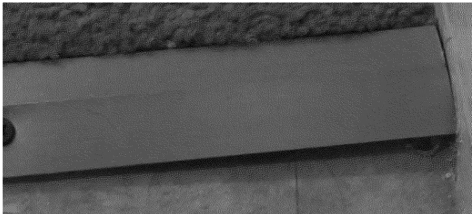
Picture 5. The M-D carpet gripper loose after fixed.
